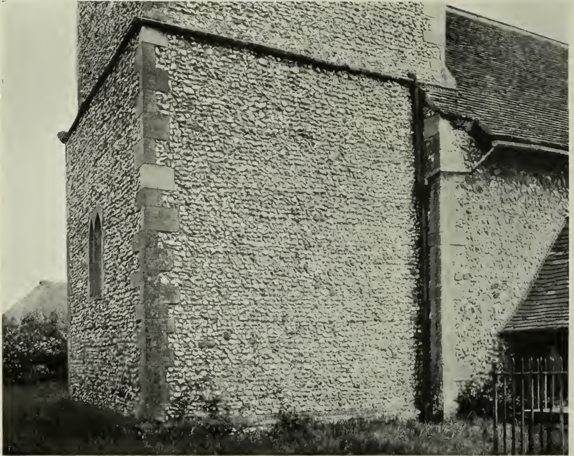
STRETHALL: PARISH CHURCH OF ST. MARY THE VIRGIN. Shewing Quoins to S.W. angle of Nave; 11th-century.
